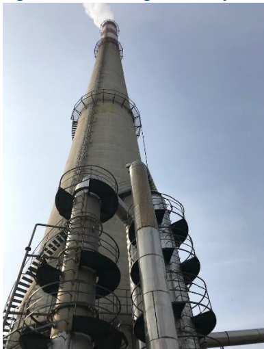
Figure 27: 120m high chimney to exhaust gas
