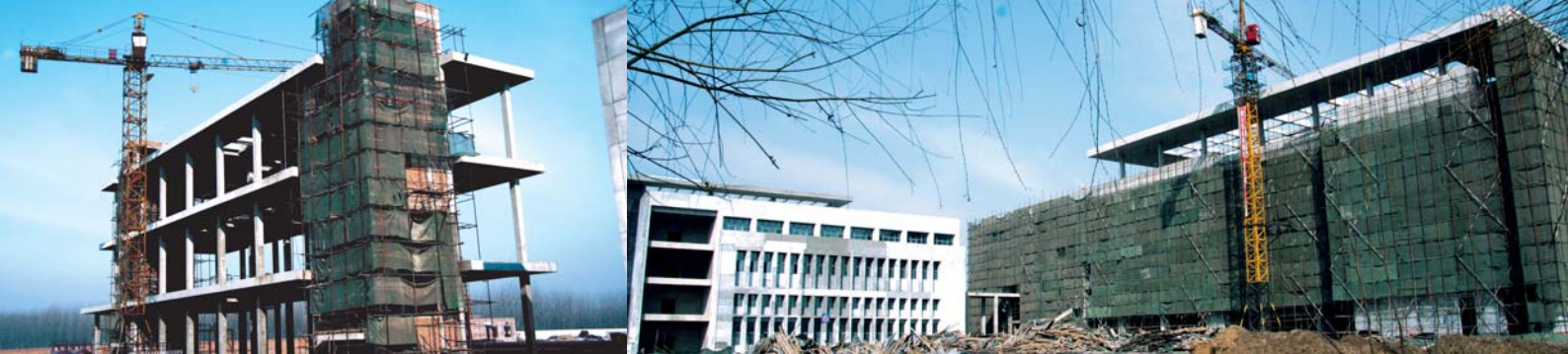
Anti-oxidant 6PPD Plant In Construction
