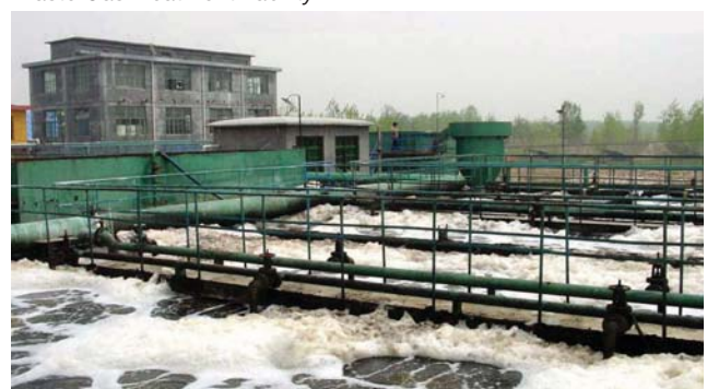
Waste Water Treatment Plant
