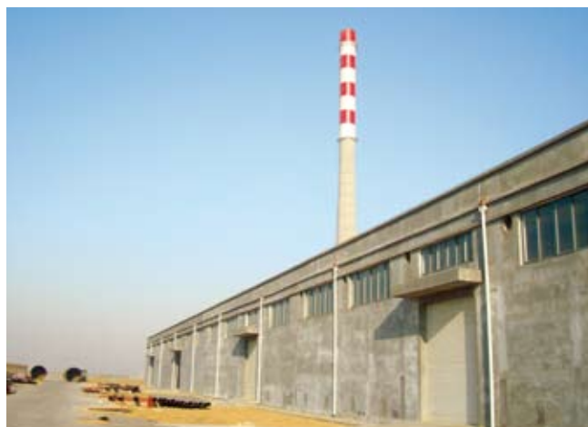
15,000-ton MBT Plant at Weifang Facility 3
