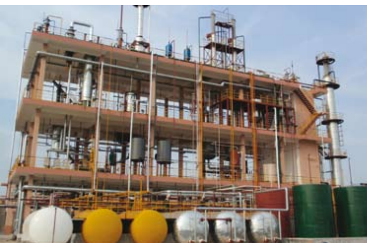
10,000-ton Anti-oxidant TMQ Workshop
