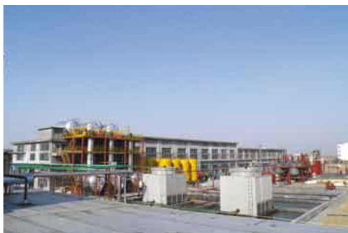
15,000-ton MBT Plant at Weifang
