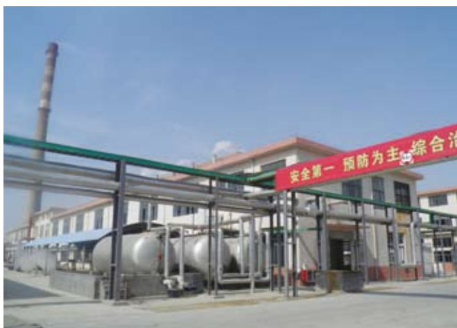
4,000-ton MBTS Plant at Weifang
