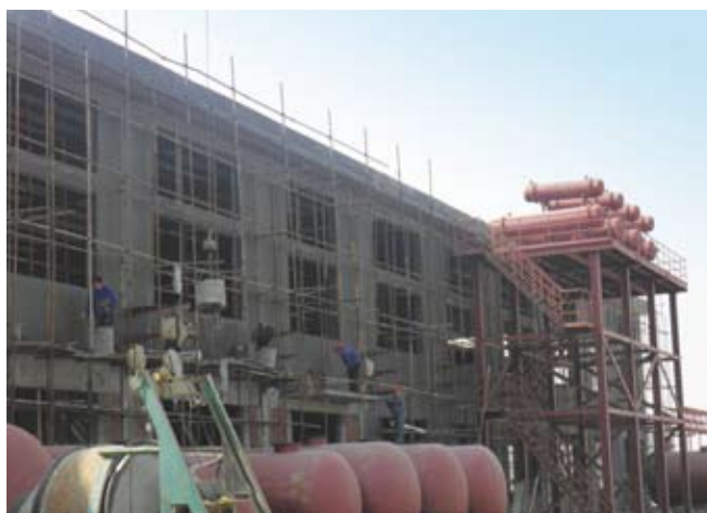
4,000-ton DPG Plant under construction at Weifang
