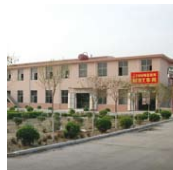
MBT Workshop at Shanxian Facility
