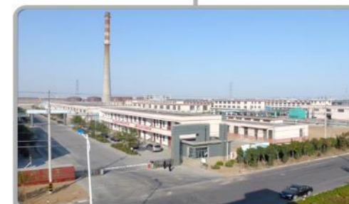
Weifang Plant • 26,000-ton accelerators
