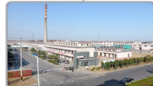
Weifang Plant • 26,000-ton accelerators
