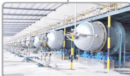
Dingtao Base • 10,000-ton Insoluble Sulphur (another 10,000-ton to be completed by 2017)
