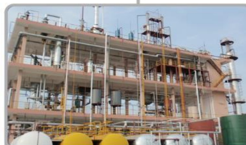
Shanxian • Home base: 116,000-ton • Sub-base-Yongshun: 10,000-ton TBBS (high-grade accelerator) expected to be completed by 2017. • Sub-base-Guangshun Heating plant: Centralised steam production
