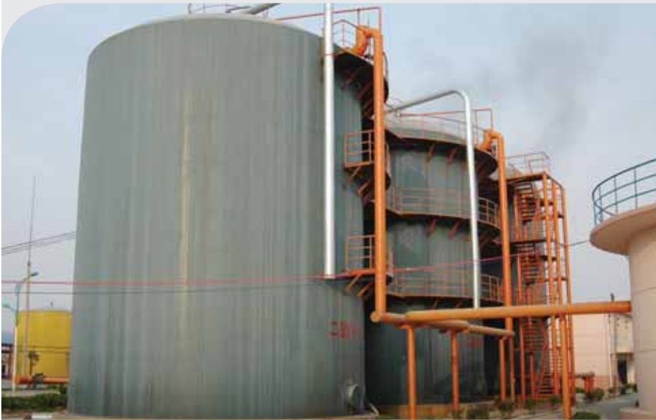
Waste-water treatment facility
