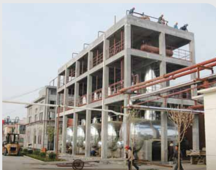
Integrated workshop under construction
