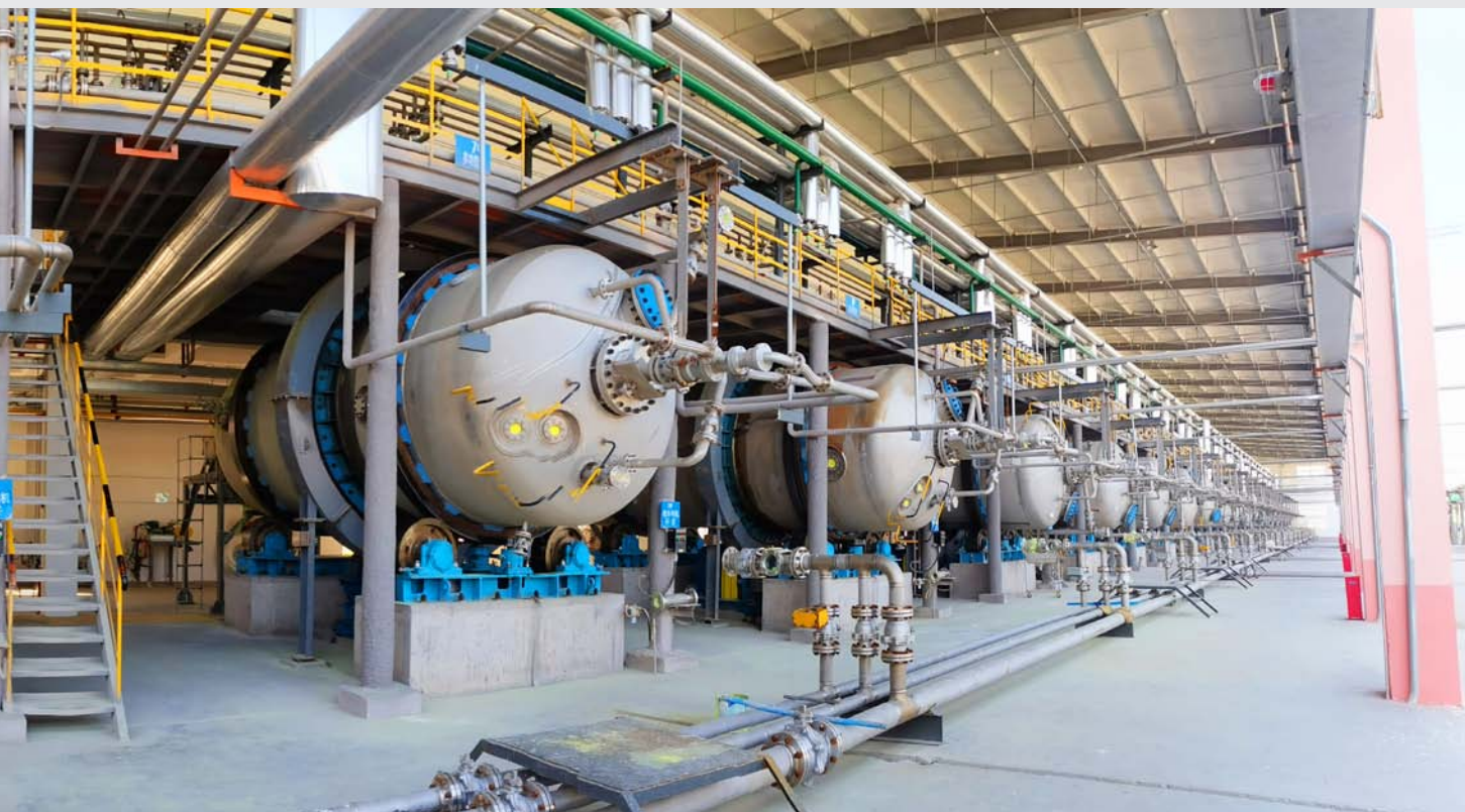
Hengshun Insoluble Sulphur Facility
